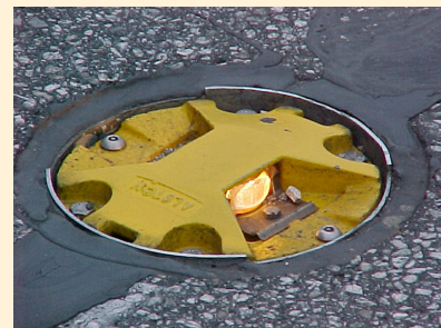
An in-pavement flashing warning light
