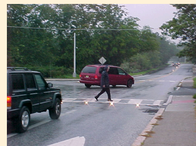
Crosswalk with in-pavement flashing warning lights installed and operating at the time of the third evaluation
