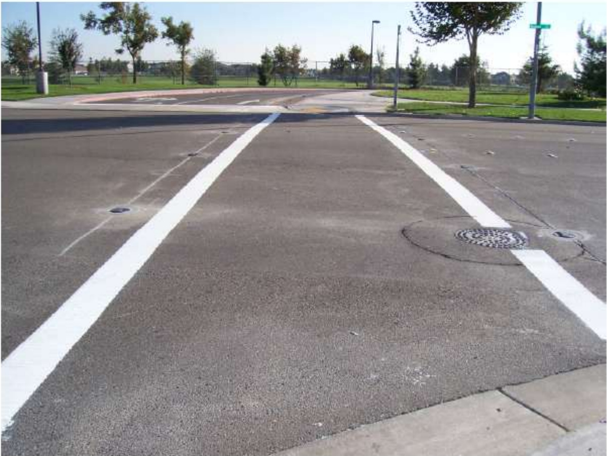
9. Fixtures Placed In Base Cans
