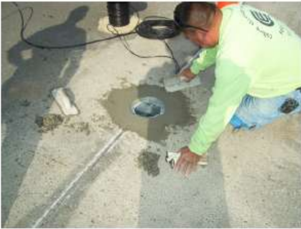
7. Base Can in Concrete
