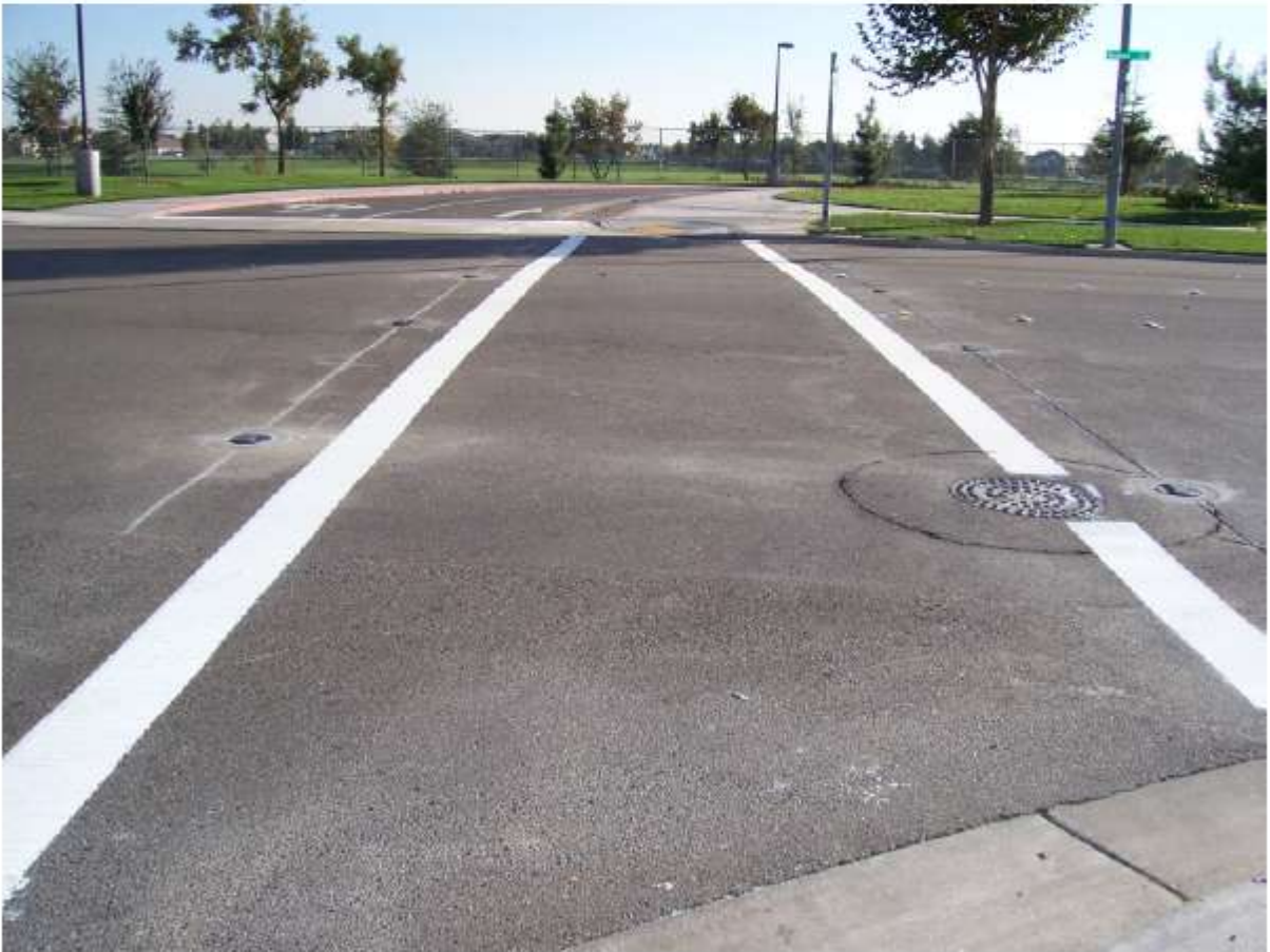
9. Fixtures Placed In Base Cans
