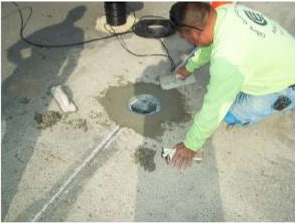
7. Base Can in Concrete
