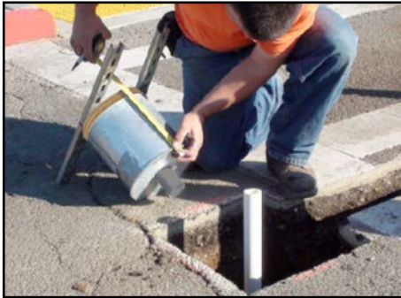
Mounting Jig Attached to Base Can
