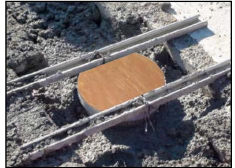
Base Can Installed in Roadway
