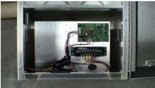
42. Final wiring is then made to the terminal block in the rear of the enclosure; the controller back panel is reinstalled, load and power cables connected, and the system's operating parameters set-up.
