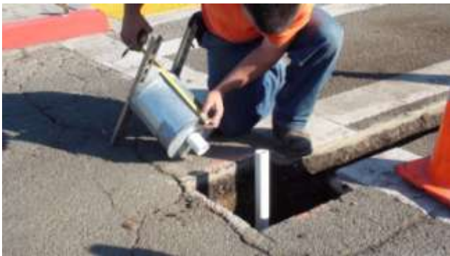
16. Base cans are then attached to drain conduit using the PVC fittings
