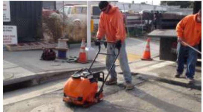
39. An asphalt compactor is used to finish the leveling and smoothing of the asphalt.
