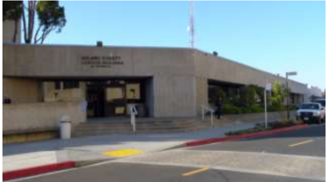
47. Solano County Justice Building
