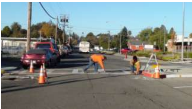
6. An outline of the trench is first sprayed onto the pavement.
