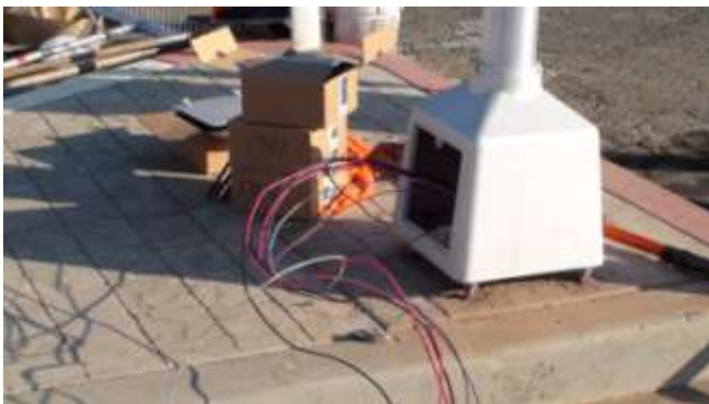
36. The process of passing the cabling through the base cans, to the pushbuttons and signs, and to the control system begins at the pole base.
