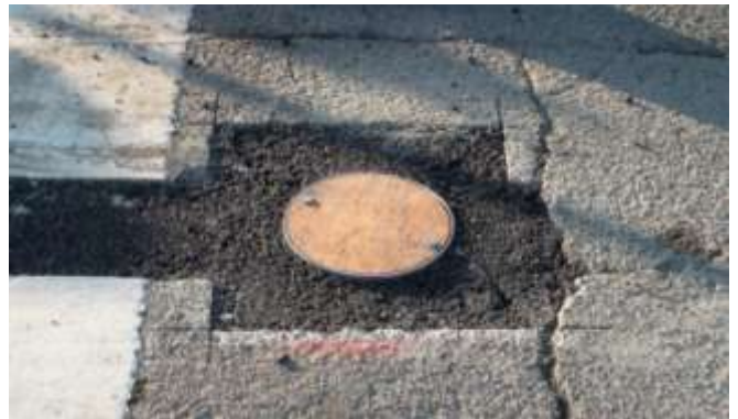
23. The mounting jig is removed, base can cleaned, and the protective plywood cover bolted onto the base can.
