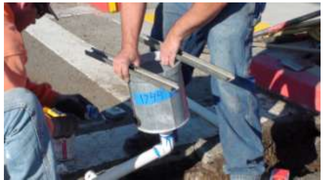
17. Base cans are then lowered into the trench.
