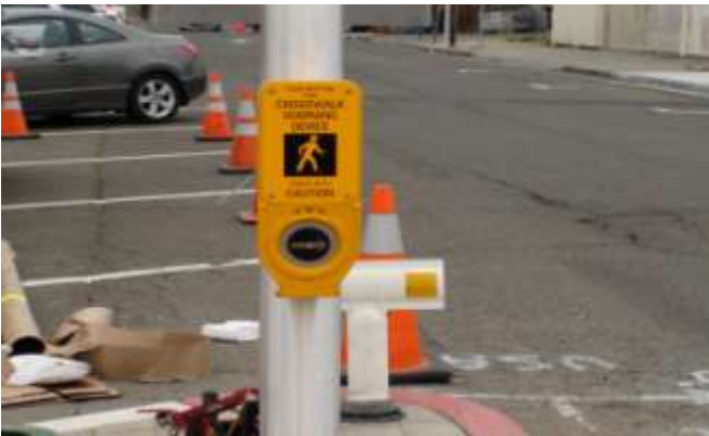
34. Cabling is attached to the terminals at the back of the pushbutton, and the pushbutton attached to the pole.
