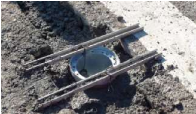
22. Quick dry concrete is generally used around the base cans; Standard concrete mix is used everywhere else.
