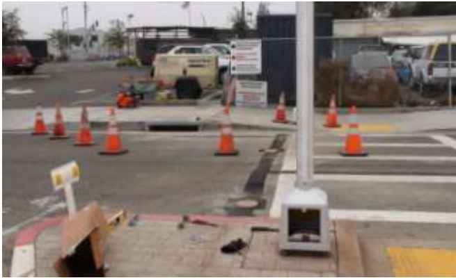
32. Pole and base are installed onto base foundation (base shown with access door open).
