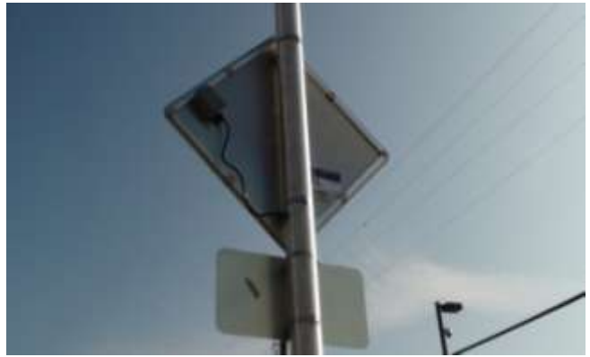
33. Flashing LED signs are installed using saddle brackets and metal straps.
