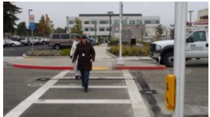
43. The solar powered TS1000 Crosswalk Warning Light System is now ready for testing.
