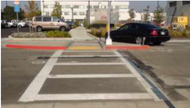
44. View of crosswalk looking towards the main parking area and Solano County building complex.
