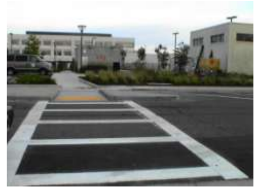
3. Crosswalk site before system installation.
