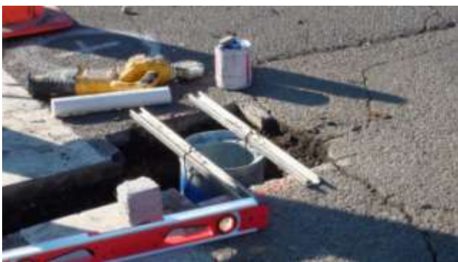
18. Dobie blocks are positioned under the conduit to prevent the base can from sinking after the mounting jig has been removed.
