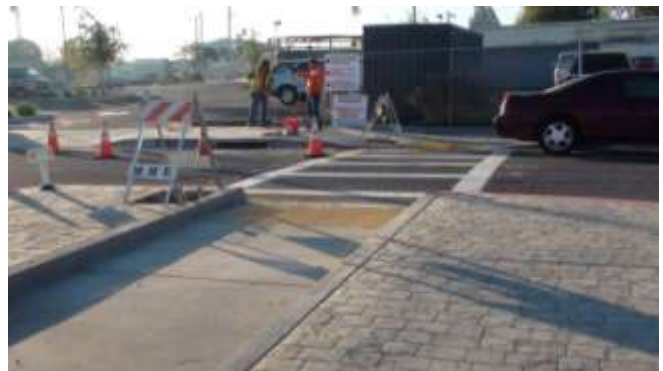
5. Site prepared and ready for trenching to begin.
