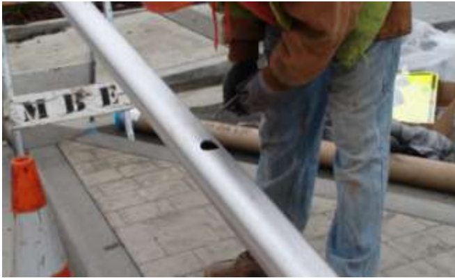
26. Access holes are cut into the pole at various locations to provide access for Electrical cabling between system components.
