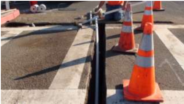
14. Drain conduit (PVC) is then installed between the base cans, and between base cans and the storm drain.
