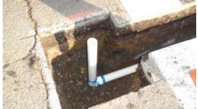
15. Drain conduit is positioned directly below the drain hole of each base can.
