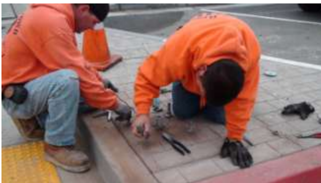
24. The treads of the L-Bolts are cleaned in preparation for mounting the pole base.
