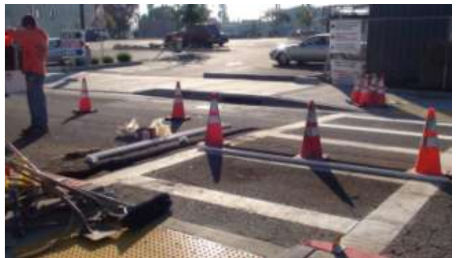
13. Drain and electrical conduit is then positioned for installation.
