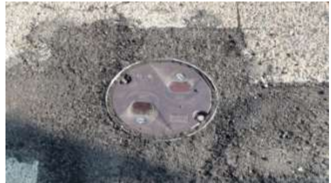
41. The plywood covers are then removed and replaced with fixtures. The fixtures are bolted to the base can. Silicon sealant is then placed into the space between the base can and fixture, providing a water proof seal.
