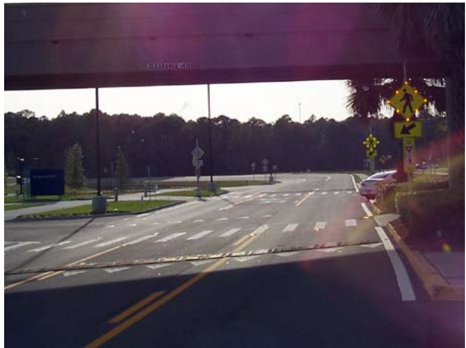
Speed humps, flashing signs, and in-pavement lighting on UNF Drive.
