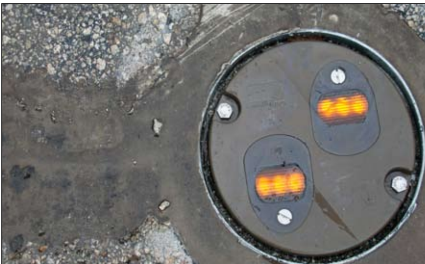
A closer look at the bi-directional TS600 LED fixture installed level with the road.
