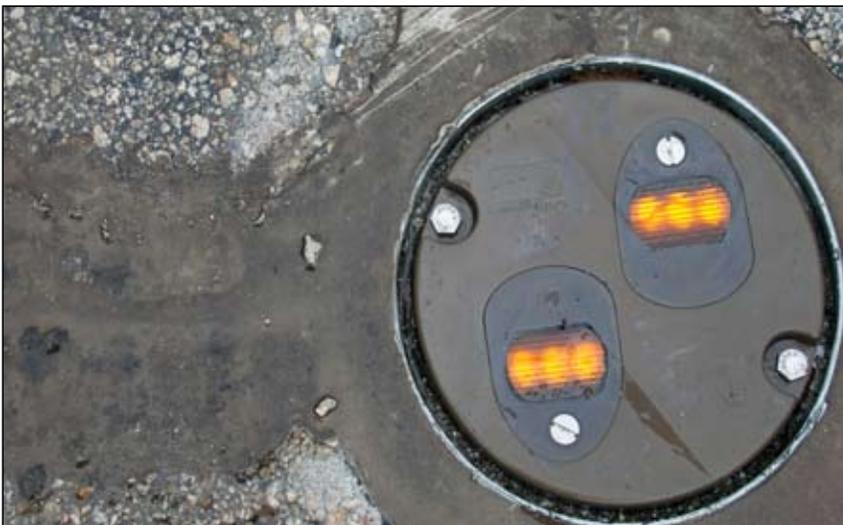
A closer look at the bi-directional TS600 LED fixture installed level with the road.
