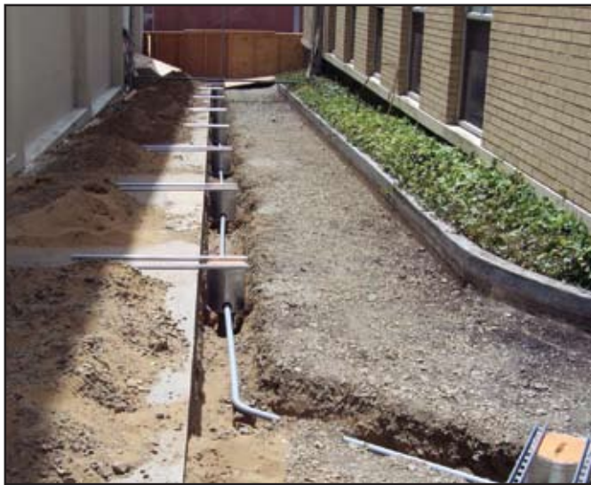
The reusable infrastructure being installed in the driveway.
