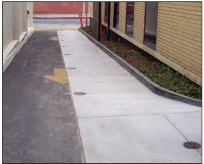
Fully-flush fixtures delineate the pedestrian path in the driveway.
