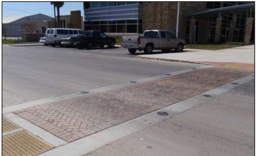
Each entrance has two Ped-X-Pads to make activation convenient for busy travelers.
