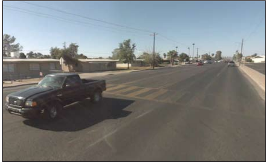
The crosswalk on the five lane road prior to installation.
