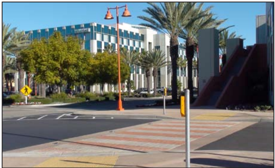
The crosswalk system enhances safety between the parking lot and shopping mall.
